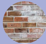
Efflorescence
